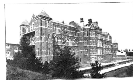
Royal Hampshire County Hospital.
